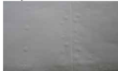
now with two layers of epoxy primer
