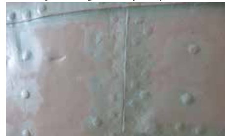
Filler has been applied
